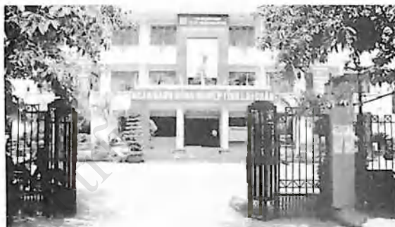
Headquarter of Lai Chau Branch of Vietnam Bank for Agriculture and Rural Development
