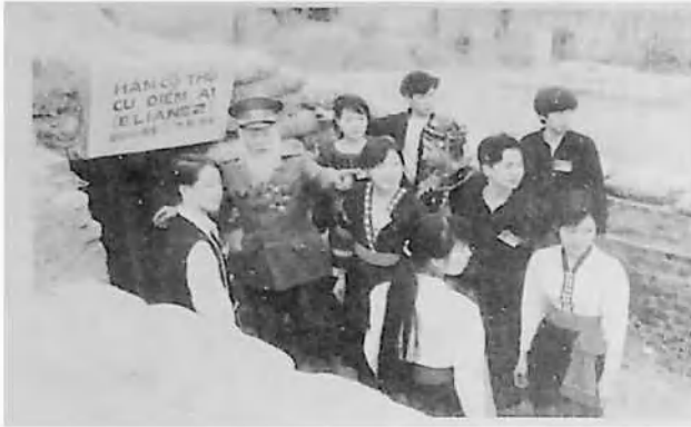
Entrance into the bunker at position A1
