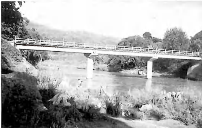
Paso bridge in Phong Tho area.
